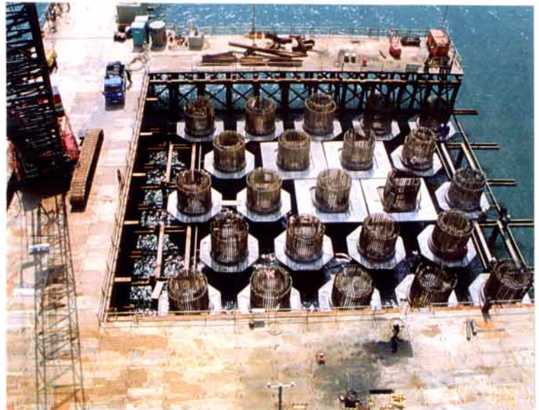
Multi-Columns with Temporary Platform
