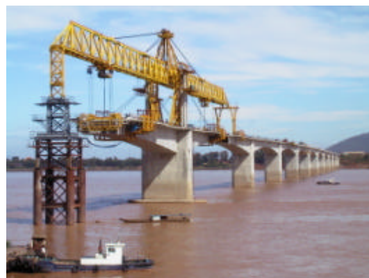
Fig. 4 Main span erection at P11
