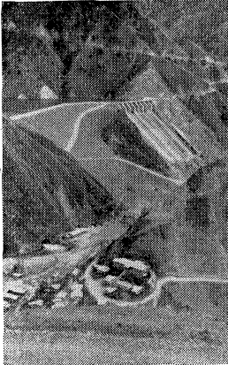
Ambuklao Rockfill Dam
