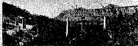
STEEL CONSTRUCTION IS POSITIONED ACROSS THE VALLEY SUPPORTING A TEMPORARY STEEL BRIDGE
