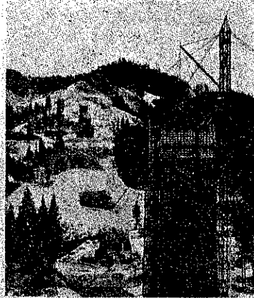
RISING PILES DRIFTED WITH REINFORCING ROSS
