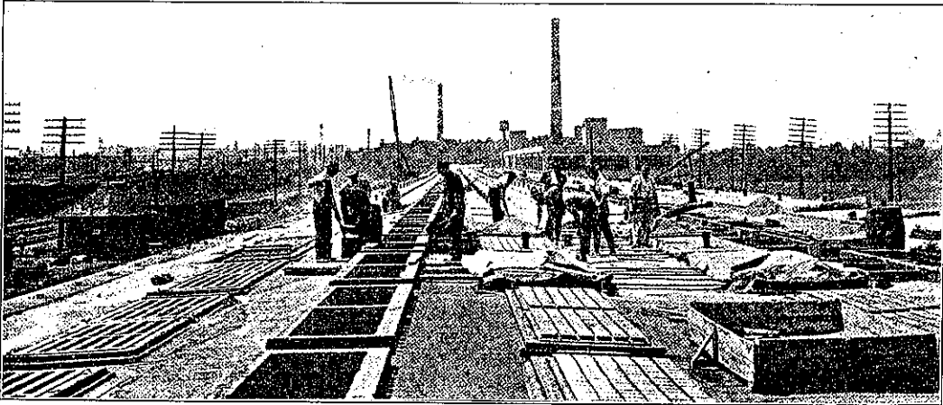
Installation of Keppler Rooflights at Curtis Street Express Building, N. Y. C. R. R., Buffalo, N. Y. Area, About 27,000 Square Feet
