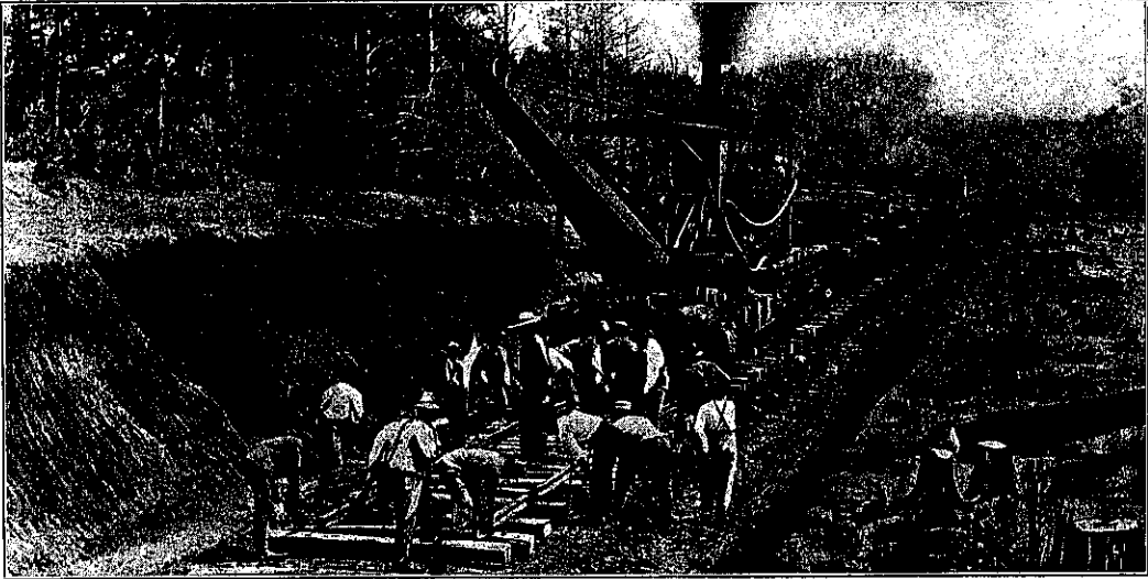
其五 Laying Track.
