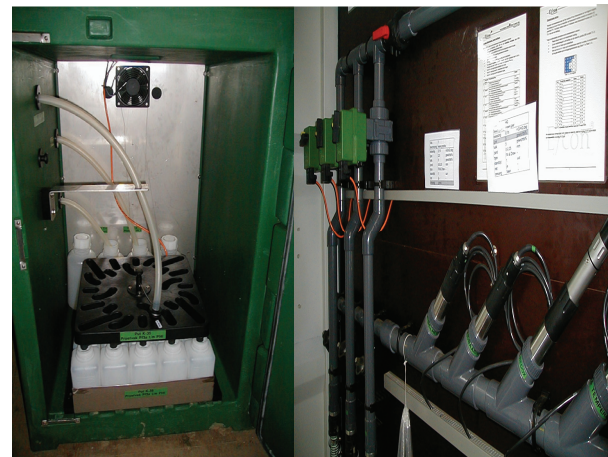
(c) Sampling device for grab samples (left) and in-situ parameters (right).
