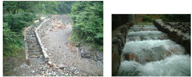
**Fig.7** Objective example of the stream type fish-way. constructed at the site of debris dam for Takizawa Dam (Japan Water Agency). The spacing and height of steps, the channel width, the side wall height and the slope are 3.5m, 0.5m, 3.7m, 0.6m and 1/10, respectively. (Courtesy Dr. H. Tatsuzawa)
