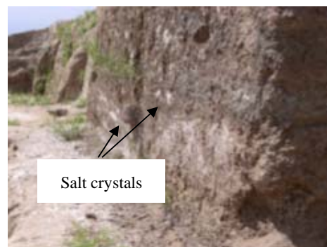
Fig.5 Salt crystallized on a historical wall
