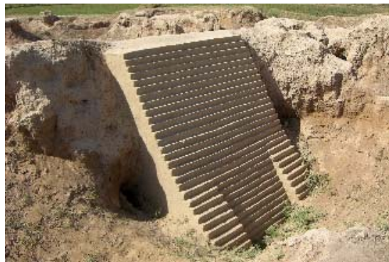
Fig.4 Support and surface cover constructed for the stabilization
