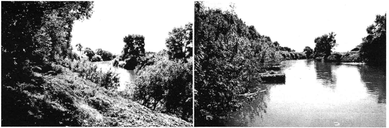
Fig. 12 Photos passed 4 years 9 months after the construction (2001.9)
