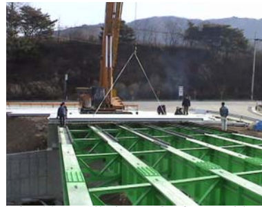
Fig. 22 Installation at Gaejung Bridge
