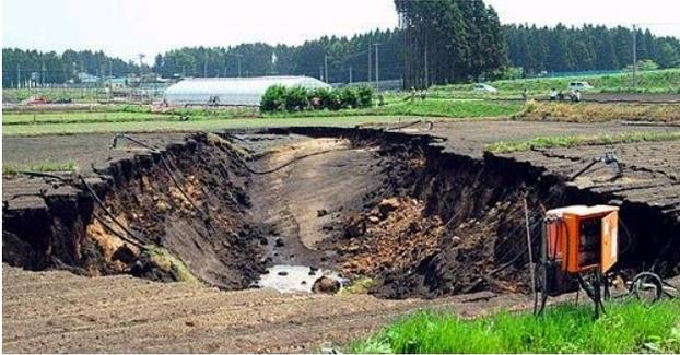
Figure 13. Surface depression due to the collapse of Shinkansen tunnel
