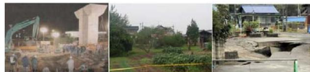
Figure 12. Formation of sinkholes and subsidence above abandoned lignite mines
