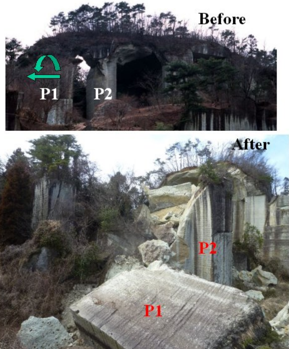
Figure 4. Totally collapsed semi-underground opening
