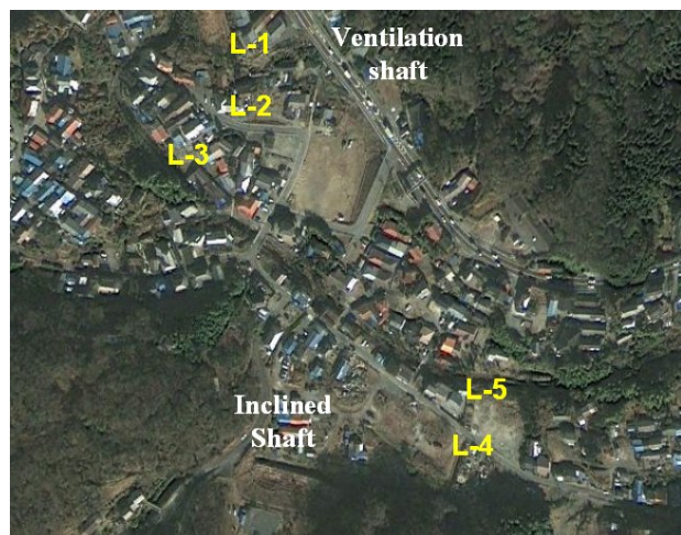
Figure 10: Locations of sinkholes at the abandoned Yoshima Coal mine
