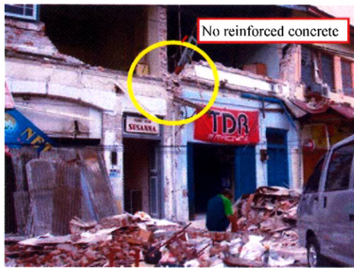
Photo 4. Example of old buildings that were built without reinforced concrete for their structures
