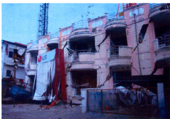
Photo 1. Example of shelter had the damage of 'soft storey' phenomenon
