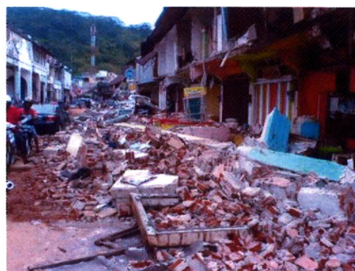
Photo 3. Example of blocked road network because of the collapsed building
