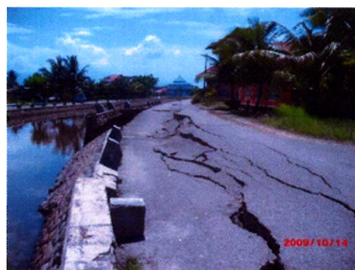
Photo 2. Example of damaged road network
