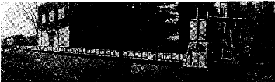
Fig. 6. General view of flood wave channel, looking downstream and water supply system.
