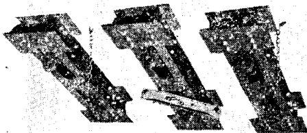
写真一2 吊 桁 Hanger beams made of 14S-T6.
