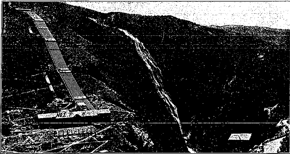
(45) Penstock, Power House, Rjukan No. 1 Development, Norway.
