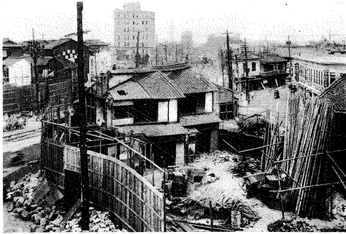
(3) 同 上——工事前の景 (3) A snap shop before construction took place.
