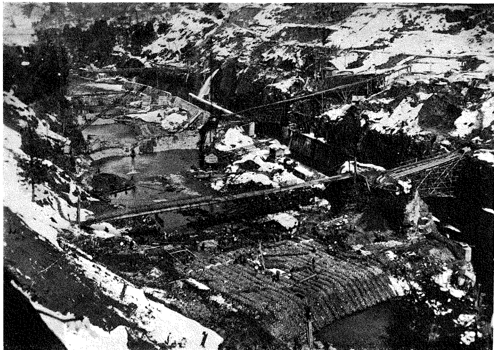
(4) In this picture, #1 and #4 coffer dam are seen. (4) 上流より見たる第一及第四假締切 (15-2-9)
