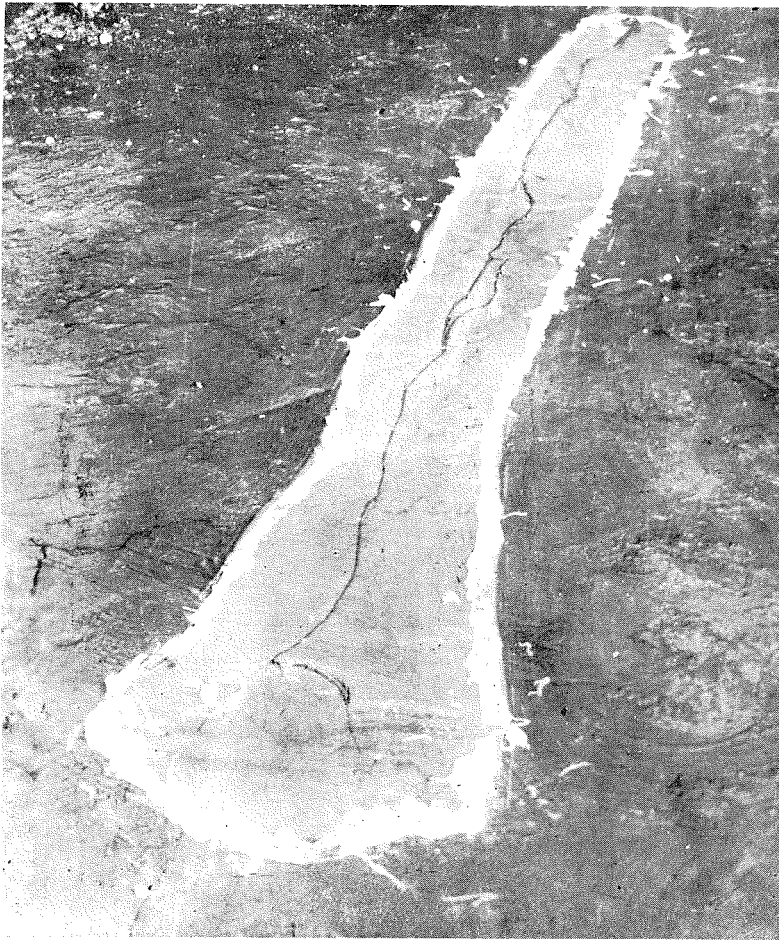
(7) Mortar is sometime ejected out of paved road after poured.
