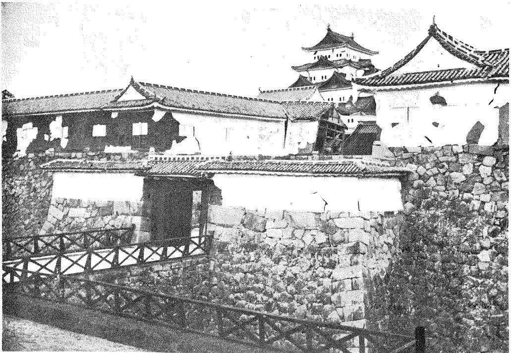
(2) A picture which shows when outside wall of the Nagoya-Castle was damaged.
