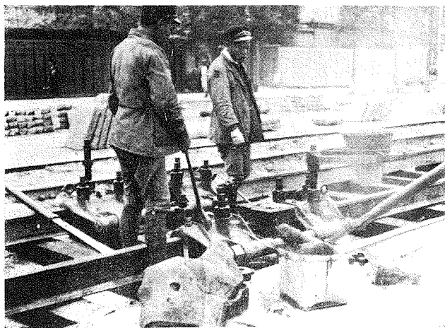
(5) Using Welding at Joints.
