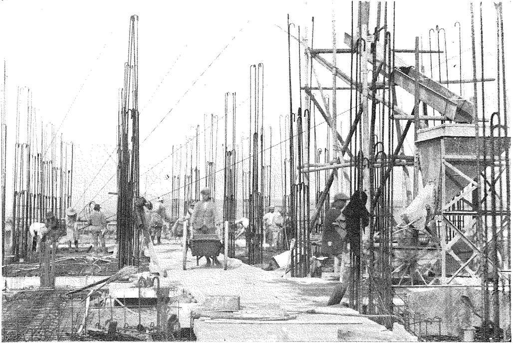
(6) Concrete Placing for Third Floor of No. 3 Ward
