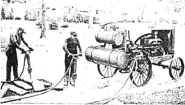
Sullivan Portable Compressor & Concrete Breakers
