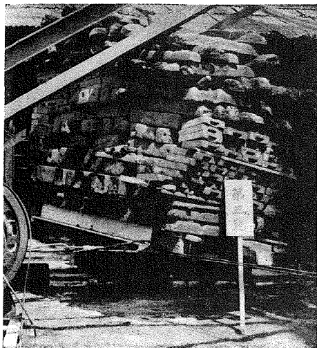
(11) Compressed the Foundation No. 3, with a Load of 67,000 lbs.
