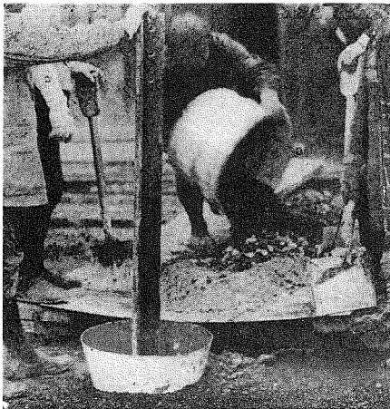
(8) Placing the Concrete in the Casing.
