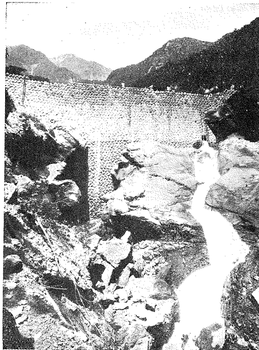
(1) 稲荷川第十三堰堤 (1) #13 Dam on Inari River, 3,250 ft. Above Sea Level. Length, 195 ft. Height, 71½ "
