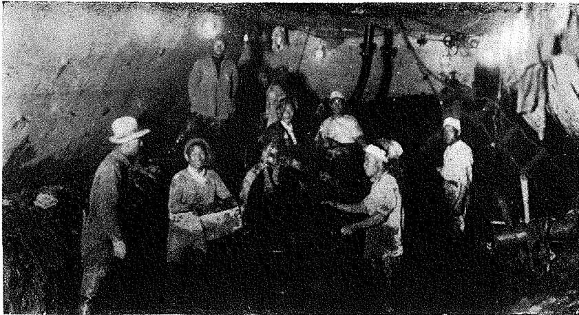
(23) 潜函底部作業室内掘鑿實況(十四年十一月二十二日) (2g) Working Men in Caisson.
