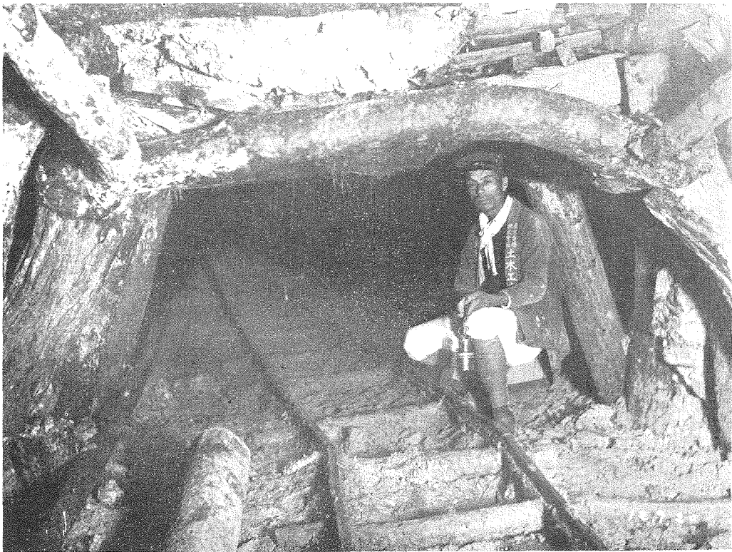
(9) Partial Collapse of Timbering in Tunnel.
