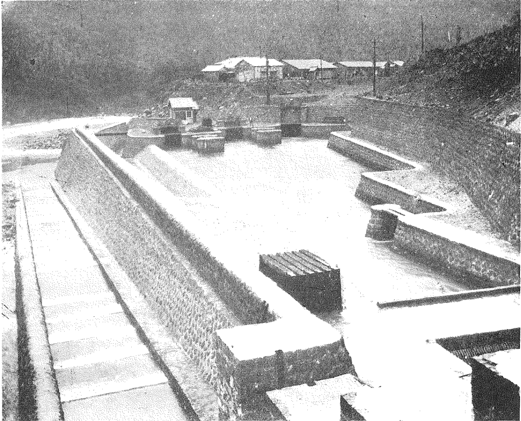
(6) Completed Intake and Sand Basin.
