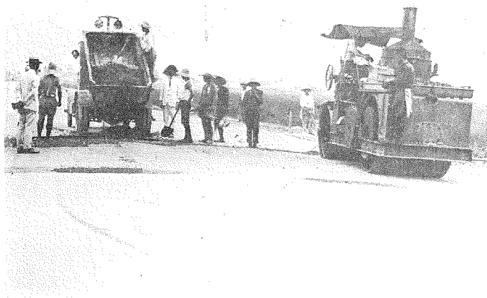
(9) Applying The Asphalt Topping.
