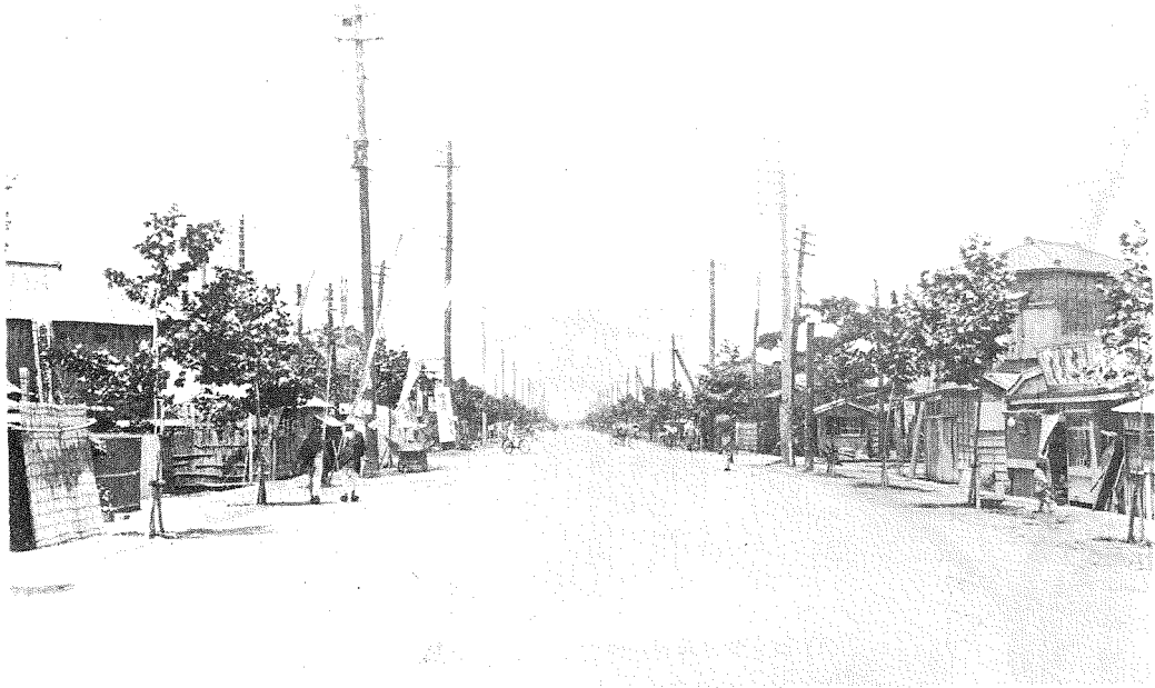
(11) The Completed Road.
