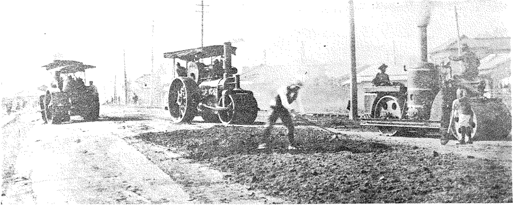
(5) 10 and 15-ton Road Rollers Working on Macadam Sub-base.
