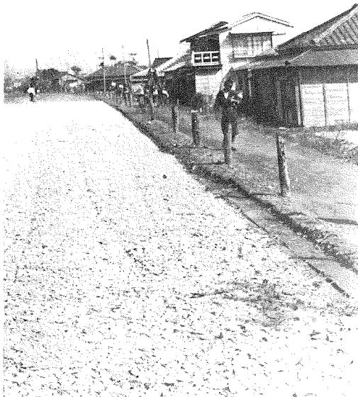
(6) Road Ready For Asphalt.
