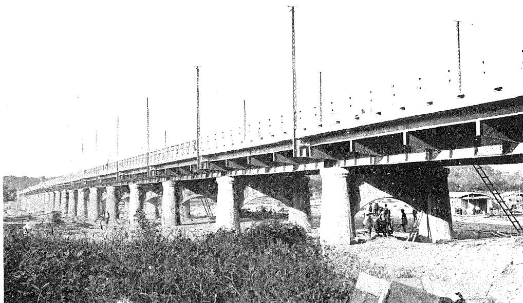
(1) 多摩川二子橋の全景 (1) General View of Futako Bridge Just Completed Across The Tama River Near Tokyo. Total Length 1,440 ft., 24 Spans. on Concrete Piers.
