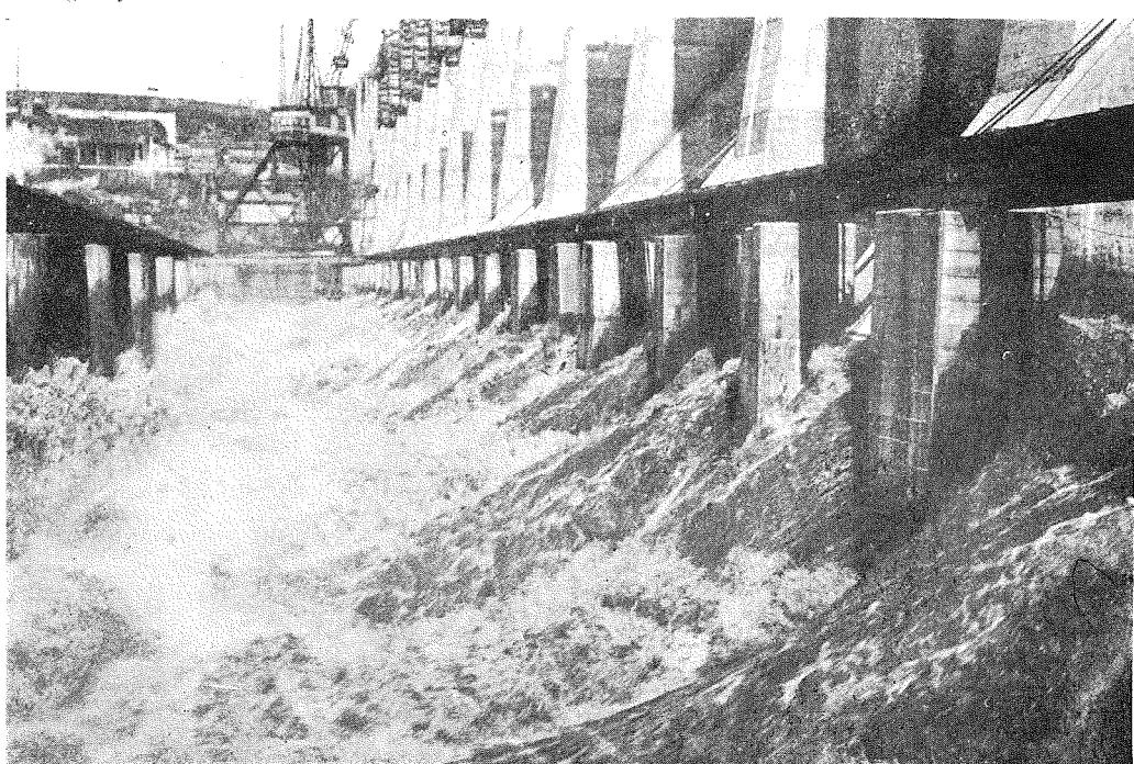
(10) メインダムの完成せざる餘水路より排水せる洪水の景 (10) Tennessee River in Partial Flood Passing Through Some of the Uncompleted Spillway Sections of the Main Dam.
