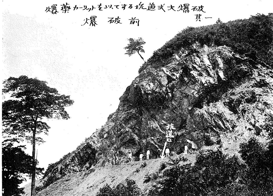
(1) Application of the Tunnel System of Blasting
