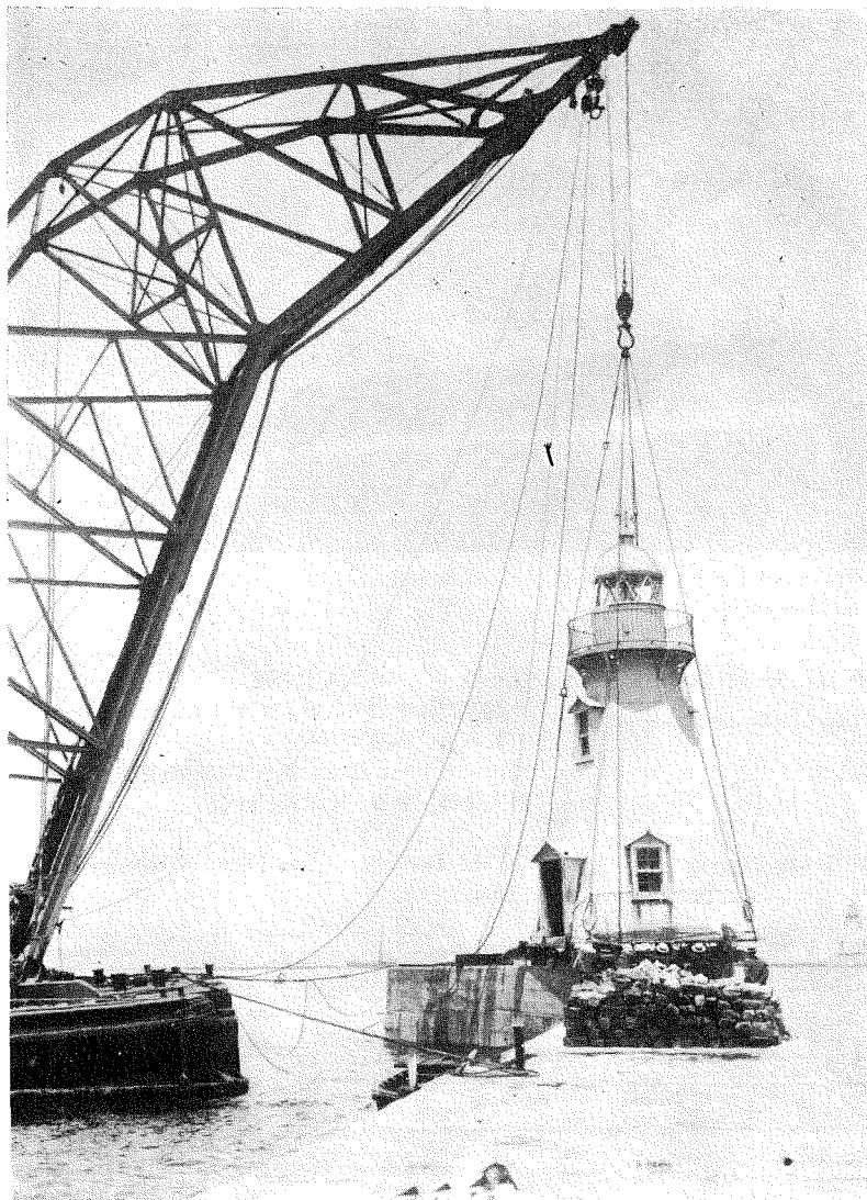
(1) At the Time of the Earthquake of 1923, the Seawall and Lighthouses at Yokohama Sank Four Meters,
