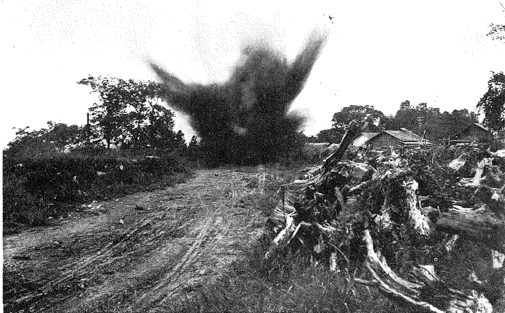
Blasting at Nagano.
