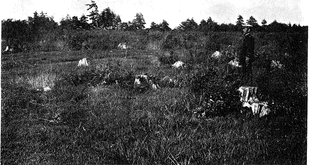
Before the Blasting at Nagano.
