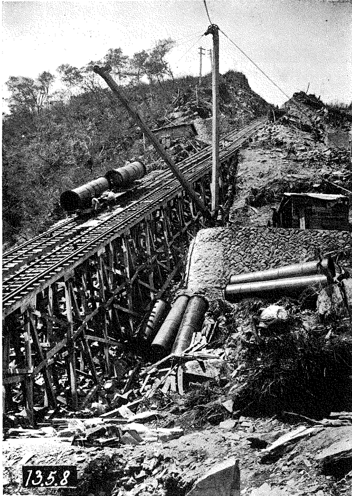
(3) 捲揚線鐵管運搬の景(信越電力) (3) Hoisting Pipes to Position.
