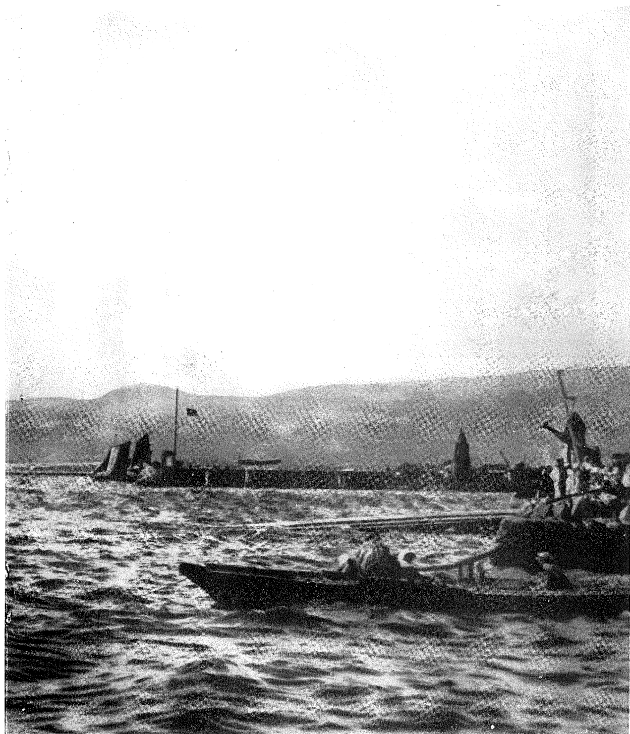
Caisson Being Launched.
