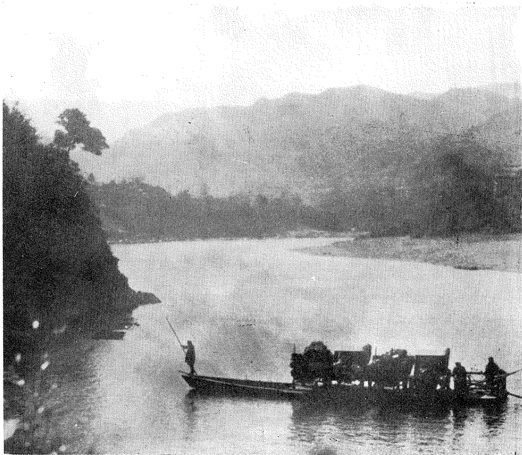
Ikeda River Ferry on Imperial Government Railway Project, near Inohana Tunnel, Yoshino River, Shikoku.
