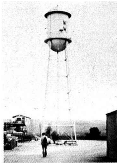
Fig. 4 Wente Elevated Water Tank
