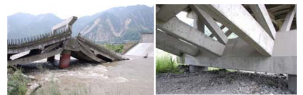
図-5 (6) P1橋脚 (右側A1)
