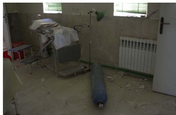
Photo 22- Falling over of a gas cylinder
