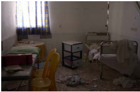
Photo 23- Displacement of equipment
