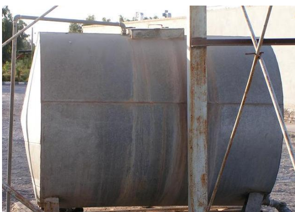
Photo 9- Water Tank 1, Aflatoonian Hospital
