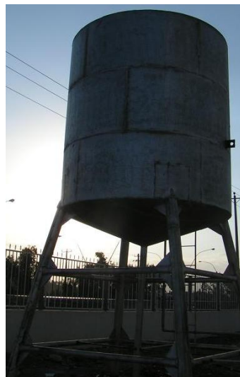
Photo 10, Water Tank 2, Aflatoonian hospital
