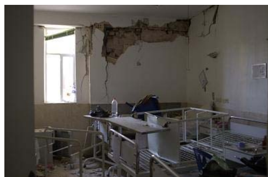
Photo 11- Topple of equipment, Aflatoonian Hospital
