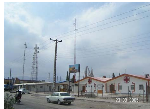
Photo 6- Prefabricated buildings installed instead of the Imam Khomeini Hospital, September 2005
