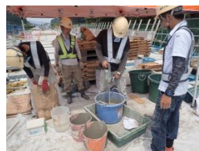
STEP7: 目地材練混ぜ
