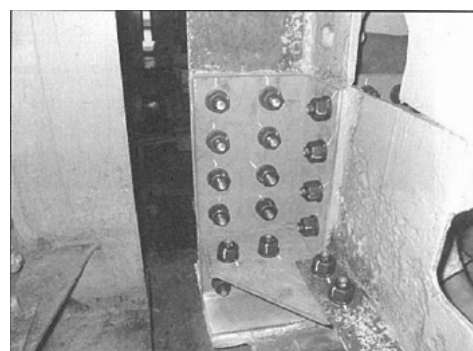
(a)鋼鉄桁橋の補修事例
