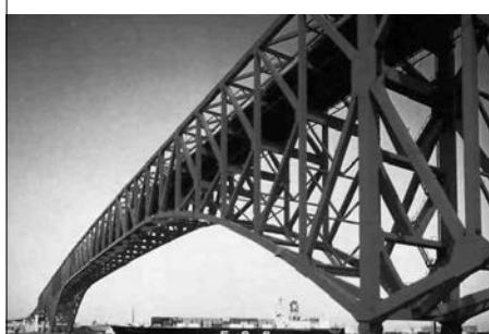
Cantilever-truss bridge with span-length 510m (3rd longest in the world)
