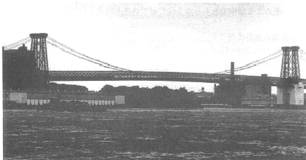
写真-1 Williamsburg bridge
