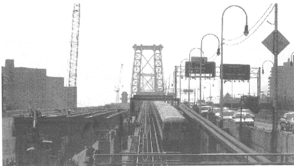
写真-2 Williamsburg bridge
