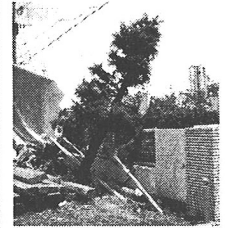
樹木や標識照明柱の倒壊
